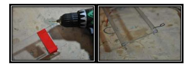
First thing to do is to figure out where to place the tray in the WTC. To do this I stick an endcap on the end and using a dry erase marker I mark a location just aft of the endcap. I like to leave a small gap just incase I want to run some wires there; the gap should be approximately  $\frac{1}{2}$ "
