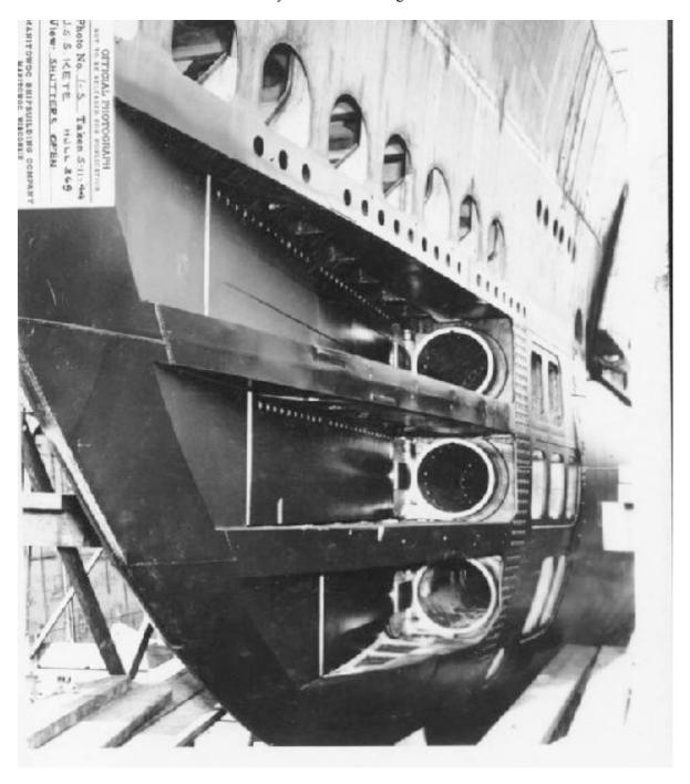
Below is an illustration of a GATO/BALAO/TENCH class American diesel-boats bow torpedo tube shutter door arrangement. How well I remember this – it was one of many illustrations in the operation pamphlet we Torpedoman studied as we learned the trade of operating and maintaining our torpedo tubes aboard the TRUTTA, a TENCH class boat.
